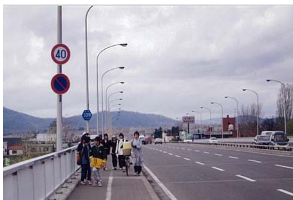
歩道幅員狭小 W=2.25m
